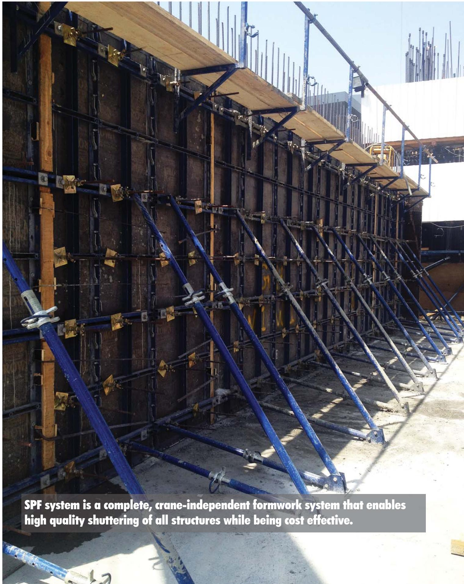
**SPF system is a complete, crane-independent formwork system that enables high quality shuttering of all structures while being cost effective.**
